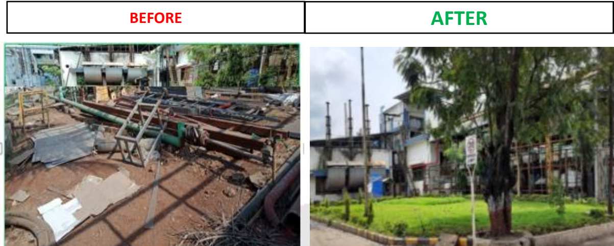
LOCATION – MC DISPATCH AREA
